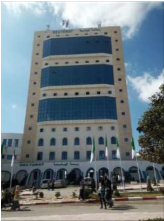
Figure 2. Case of study office building.
