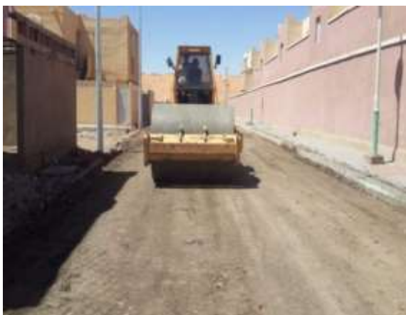
Figure 4. Compacting of RTS.
