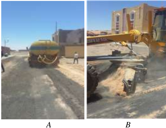
Figure 3. A: Water Spraying, B: Mixing.
