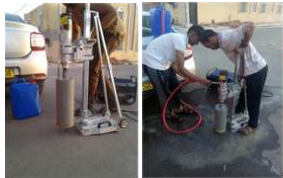
Figure 17. Coring concrete pavement layer.
