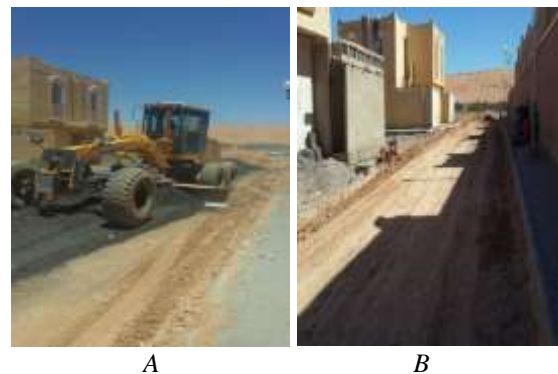
Figure 2. A: Soil stripping, B: materials spreading.
